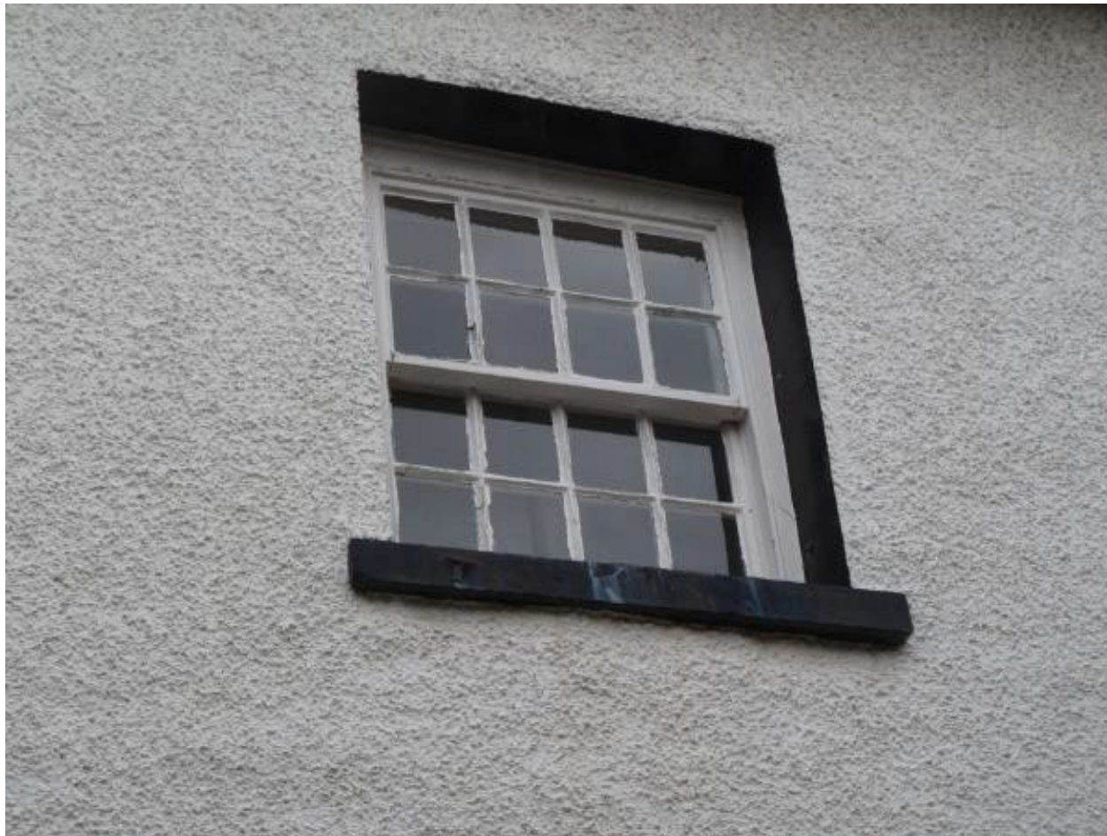
Figure 30: Historic windows and other features should be retained.
