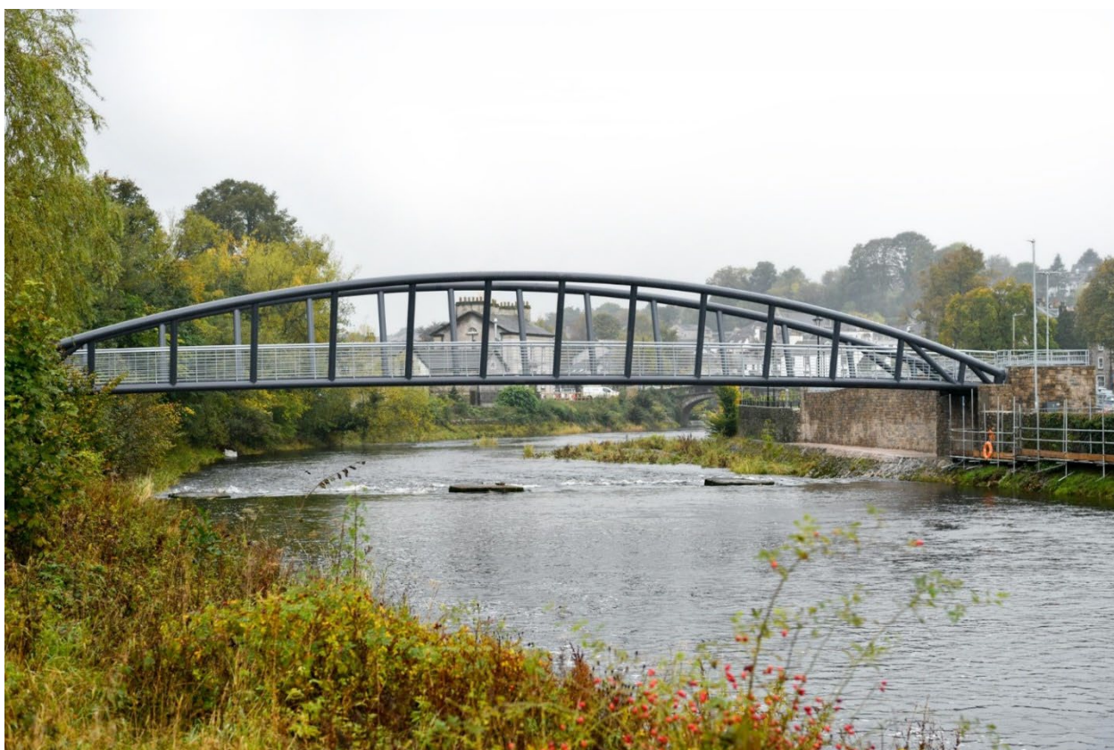
Figure 1: Photograph of Gooseholme Bridge, Kendal
