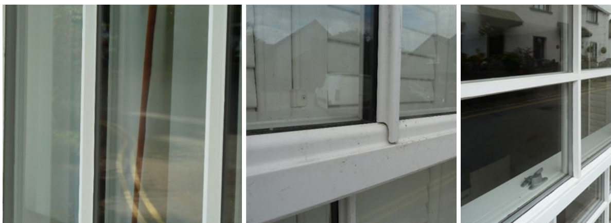
Figure 5 Black seals makes double glazing extremely obvious, and spoils an otherwise well-designed PVC window. Centre: Obvious double glazing with a prominent black seal. Plastic glazing bars appear very obvious with a gap at the bottom where they attach to the meeting rail. This would not be seen in a traditional timber sash. Right: the panes have an unusual horizontal emphasis. Sash window panes usually possess vertical proportions. This is exacerbated by the poorly detailed glazing bar profile which is overly thick and not reflective of the elegant slender proportions of C18-C19 sashes.
