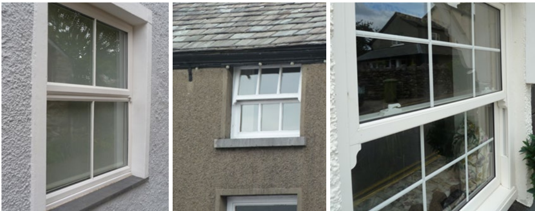
Figure 4 Top hung casements, in plastic and timber (left and centre), protrude from the face of the building when open and are a poor imitation of a traditional vertically sliding sash. When closed there is a horizontal line between the meeting rails and the added horn (which counterbalances the weight of a traditional sash) is inauthentic and draws attention to their poor design. Right: Double glazed PVC with applied plastic strips to imitate glazing bars creates a flat face to the window.
