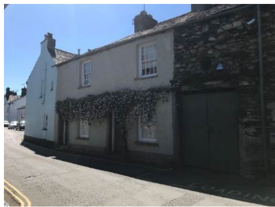
Figure 13. Chestnut Cottage, 2019. Roof covering, chimney stack, roughcast render, joinery and rainwater goods are all appropriate and in keeping with the period of the property.
