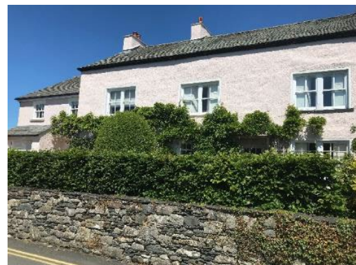
Figure 19. Hartwell House, 2019. Slate roof, roughcast render, chimney stacks, timber sash windows.
