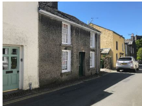
Figure 17. Stonecroft, 2019. Two storey double-fronted house, C19. Retains single glazed windows, chimney stack and roughcast render.
