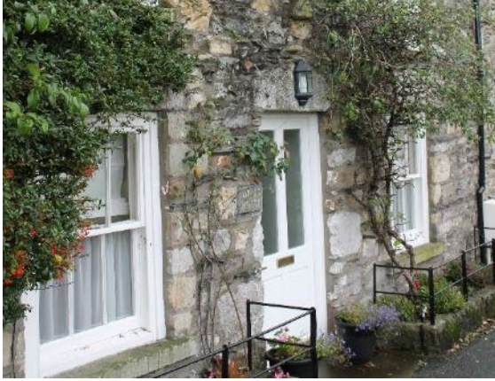
Figure 10. Wells House, 2014. Timber door to frontage.
