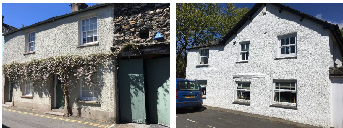
Figure 26. Original sashes on Cavendish Street (left) and low quality replacement windows (right)
