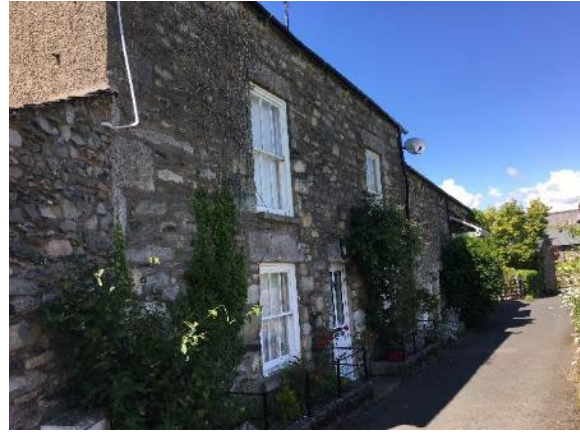
Figure 11. Wells House, 2019. Timber door has been replaced with white upvc door, under permitted development.
