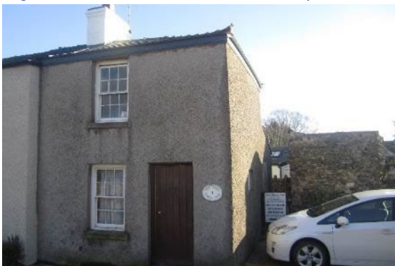
Figure 8. No. 2 North View, 2014. End terrace cottage with single-glazed sliding sash windows.
