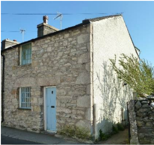
Figure 4. End Cottage, The Causeway in 2014. Original windows and door intact.
