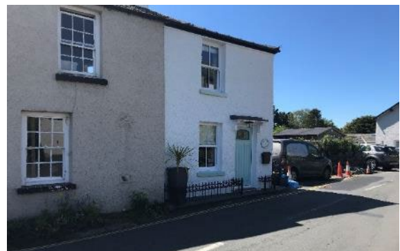
Figure 9. No. 2 North View in 2019. The small-paned windows have been removed and the door replaced. Railings and a canopy added to the frontage, also affect the unity of this group of cottages in the conservation area.
