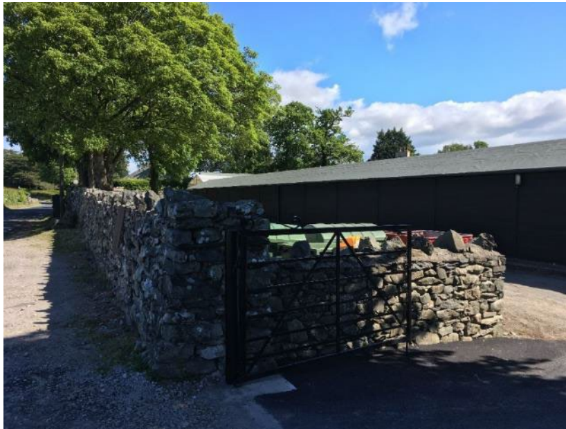
Figure 32. Cartmel Racecourse Stables, Park View
