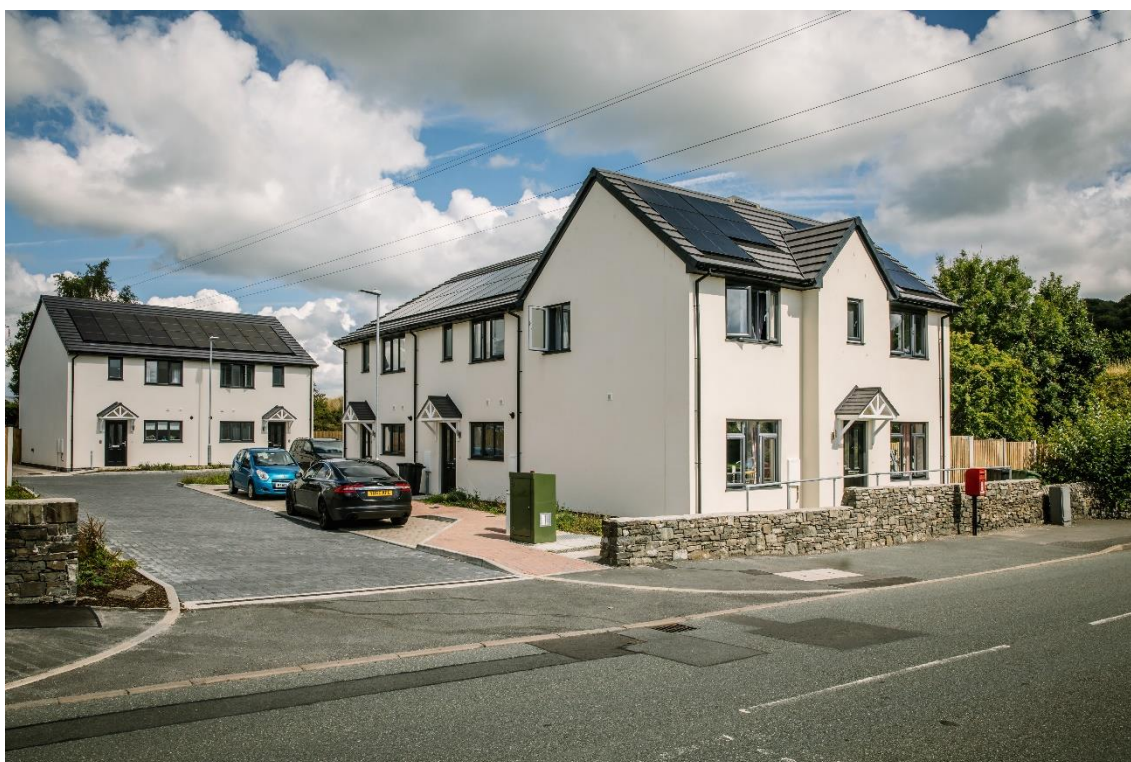
Figure 1: Parkside Road, Kendal affordable housing scheme
