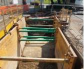
EA contractors replaced the existing masonry arch culvert within the car park with a precast concrete box culvert. This ensured the culvert remains serviceable for the next 100 years and will reduce the risk of flooding.
