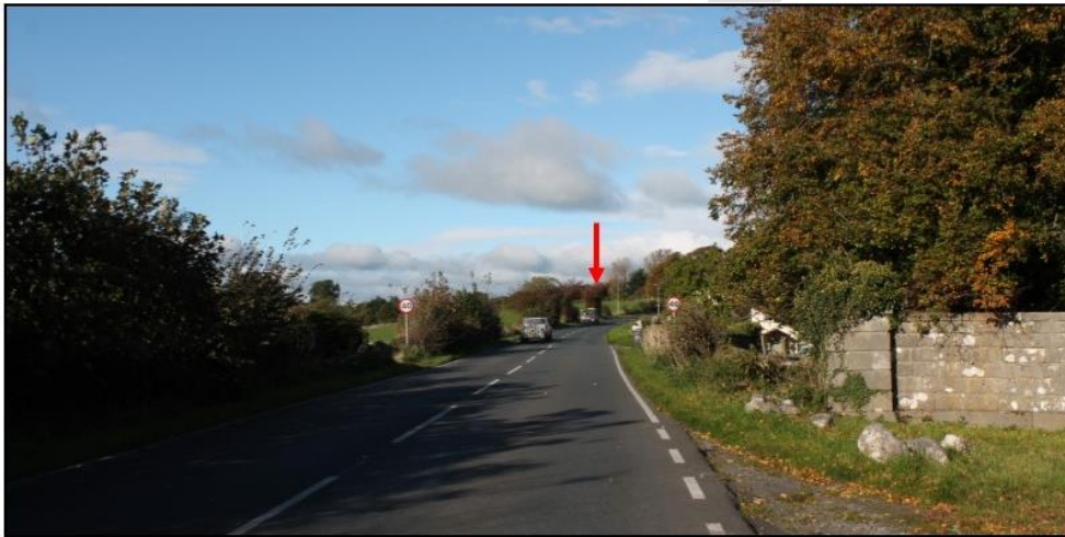
Figure 5: Site on approach from south along the A6070
