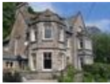
Former Residential School, Woodlands & Low Slack, Queens Road, KENDAL, Cumbria
