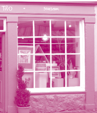
The whole window surround in this shop in Ulverston is constructed from stone
