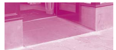
A good example of a slightly ramped door threshold which will aid access for users with limited mobility
