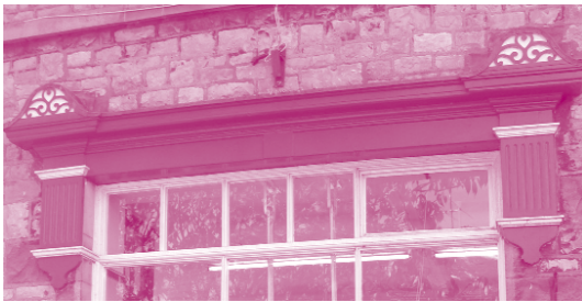
An unusual, truncated, pilaster design around an early twentieth century shop window in Kirkby Lonsdale
