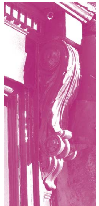
Intricately carved timber console bracket in Kendal
