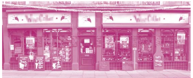
Shopfronts showing an excessive use of window stickers and sandwich boards can detract from the shopfront and limit the opportunity for easy window shopping
