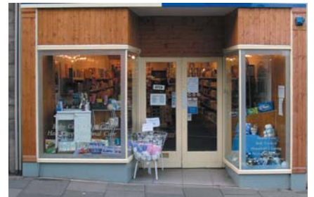
The use of unpainted timber is rarely sympathetic or harmonious in historic areas
