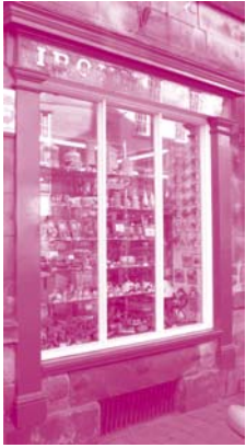
Large areas of glass can be broken up through the use of mullions, as here in a shopfront in Kirkby Lonsdale, or with horizontal transoms
