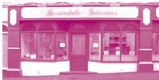
A recent shopfront with poorly proportioned pilasters, which try, unsuccessfully, to imitate those in traditional designs: here the pilasters are far too wide, have unevenly sized divisions, and fit awkwardly to the fascia and transom lights
