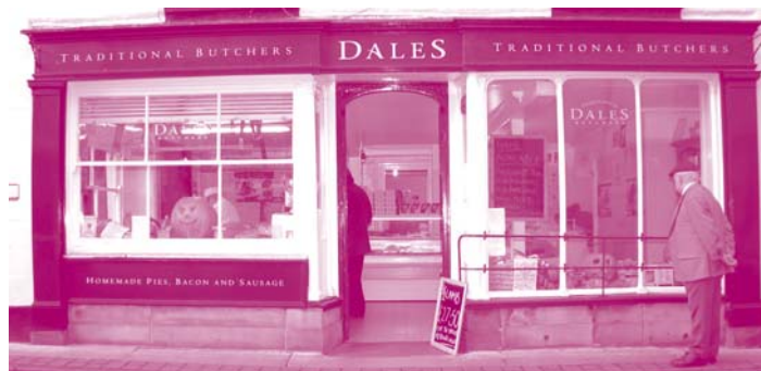
Characteristically asymmetrical arrangement for a traditional butchers shop with an opening sash window on one side that allowed the goods to be better displayed
