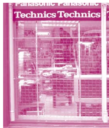
The combination of toughened glass with internal lattice grilles can provide better security and still allow window-shopping to take place out of hours
