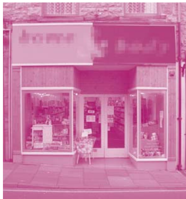
An ill thought out shopfront, with an excessively tall fascia and a lack of any cornice, help make this shopfront appear uninspiring in design terms
