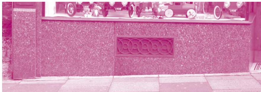
Polished granite stallriser in Grange over Sands
