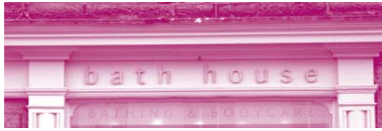
Attractively scaled, well moulded cornice and narrow fascia on traditional shopfront in Kirkby Lonsdale, with effective modern lettering added
